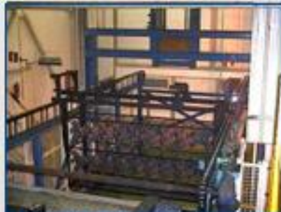
3 Painting installations by cathoresis (KTL, incl. silicates removal)
